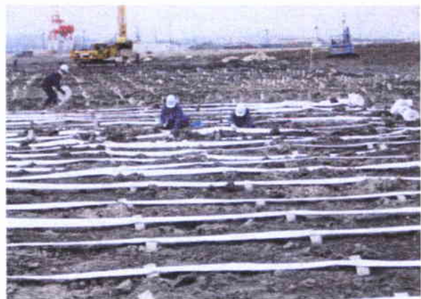
Installation of SB Drains along with CN Drains
