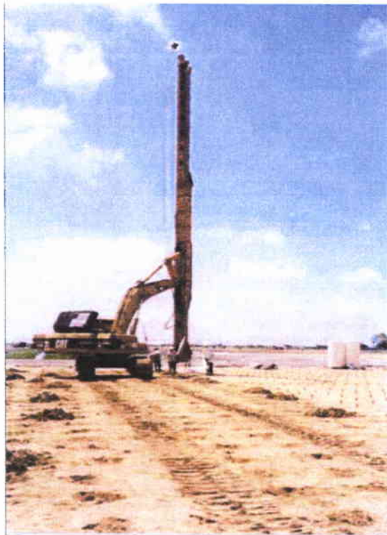
Typical PVD Installation on Ground
