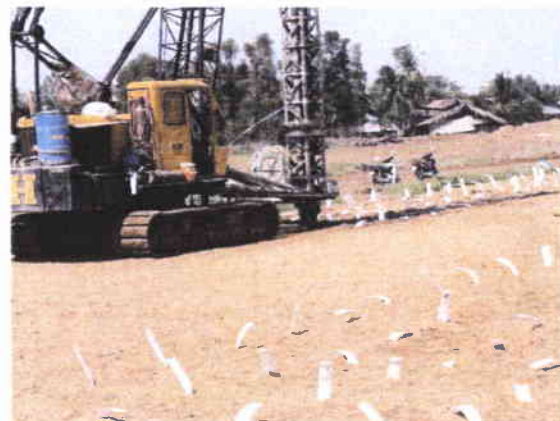
PVD Installation in Vietnam
