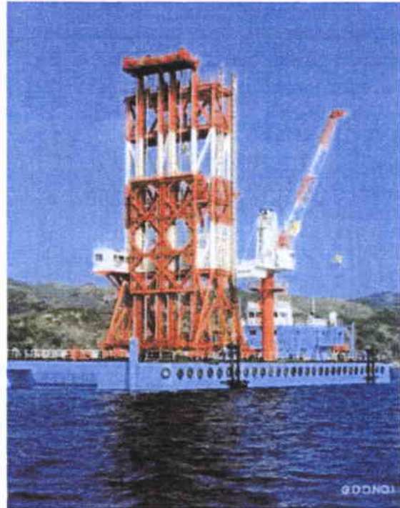
Offshore PVD Installation in Japan
