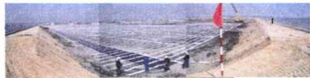
Installation of SB drains in Confined area
